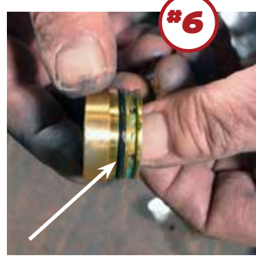
Replace the O-Rings on the seal retainers.
